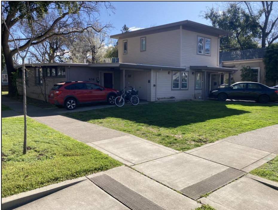
West façade of subject property with 2017 two-story addition, view facing southeast (ESA, 2024).
